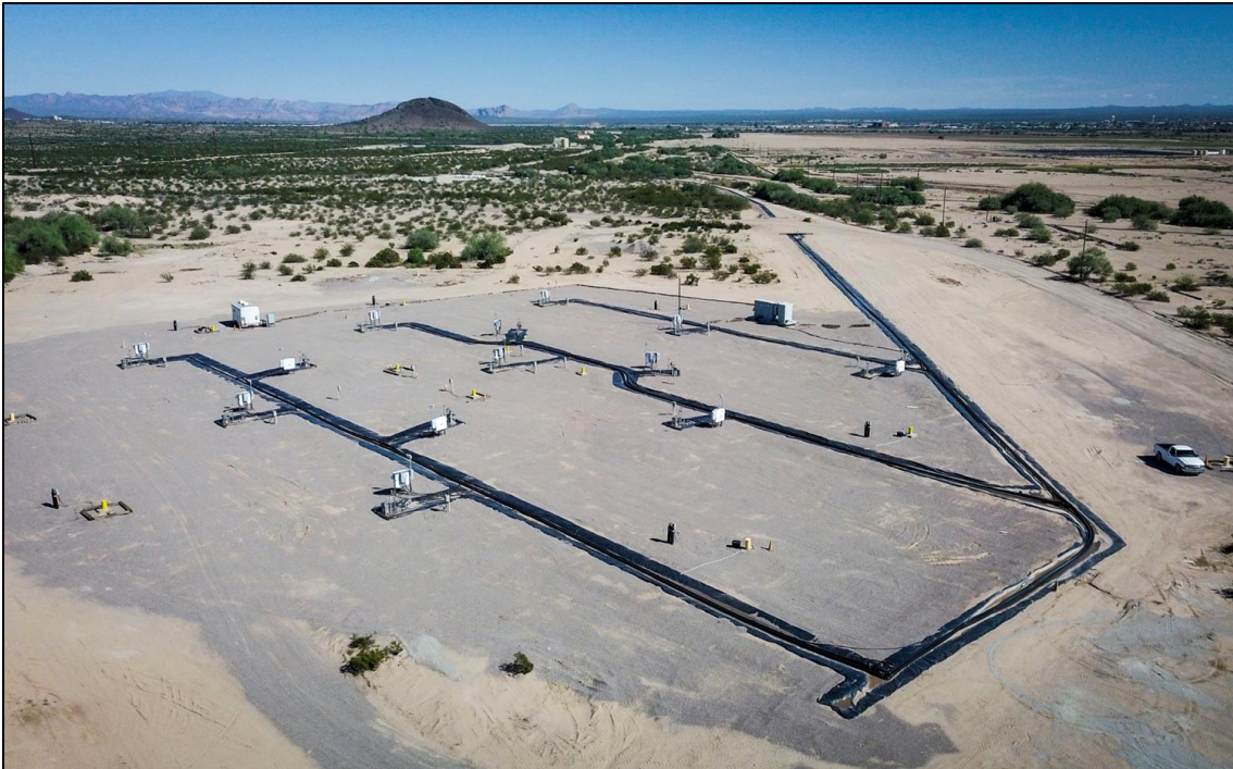
Figure 13-8: Aerial View of PTF Well Field
